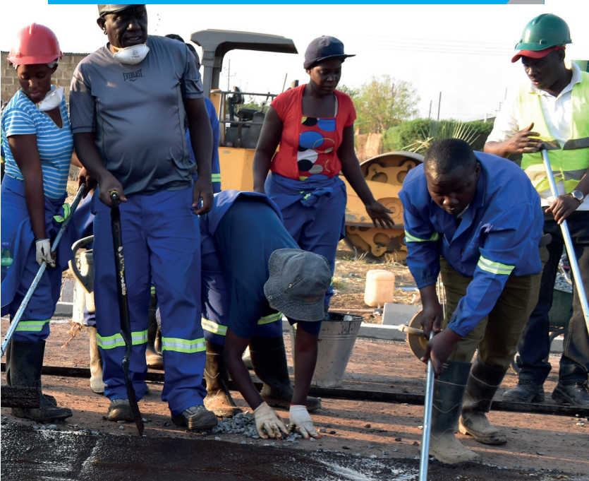
Contractors demonstrating the cape seal technology on the Lubombo Road
