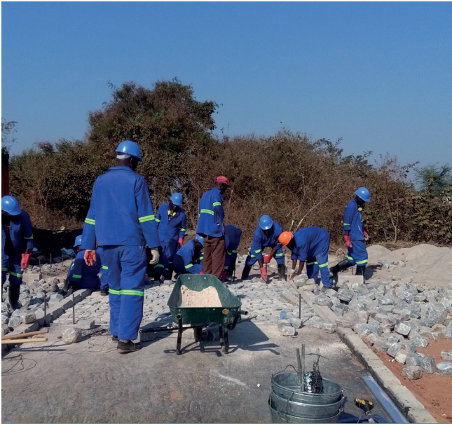
Pavers laying cobbles during demonstration.
