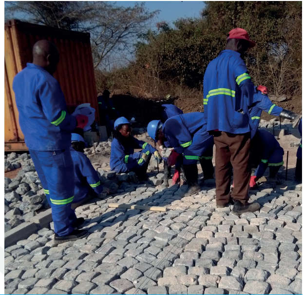
Pavers laying cobbles during demonstration.
